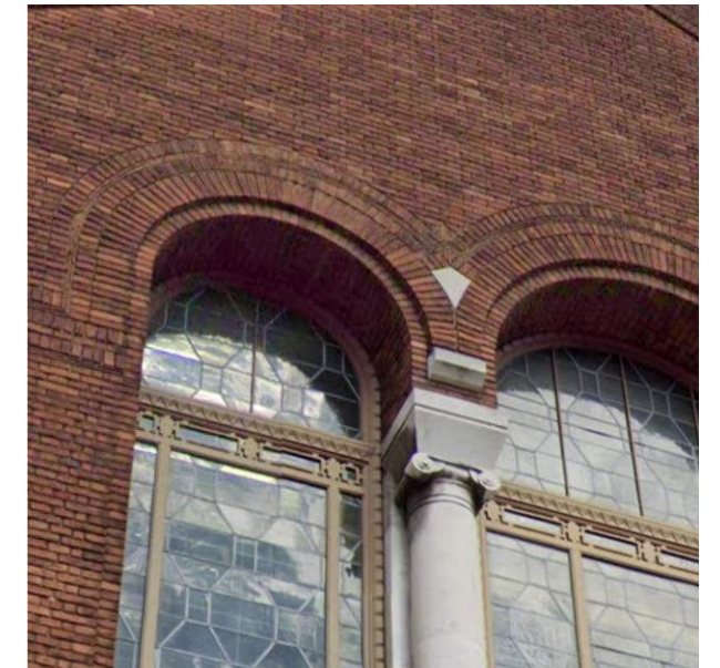
Second Church of Christ Science: Brick details to arches
