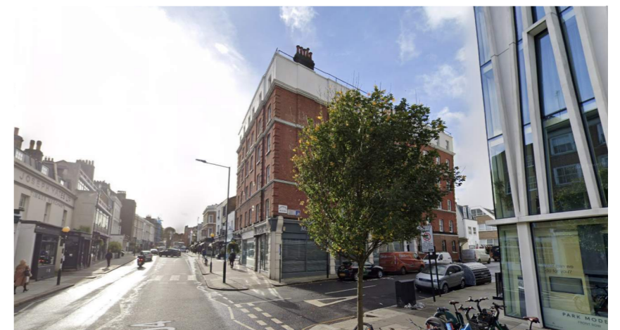
Fig. 3.98: Corner Mansion Block Condition: Campden Hill Mansion to Kensington Church St.
