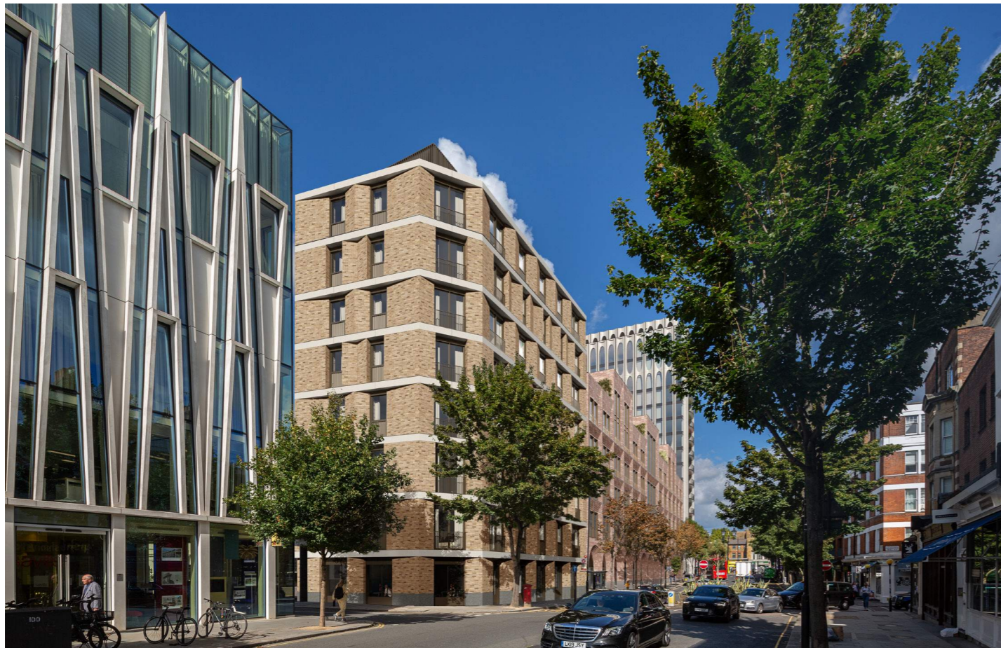
Fig. 3.95: QRP 3 Illustrative View from Kensington Church Street looking towards Notting Hill Gate
