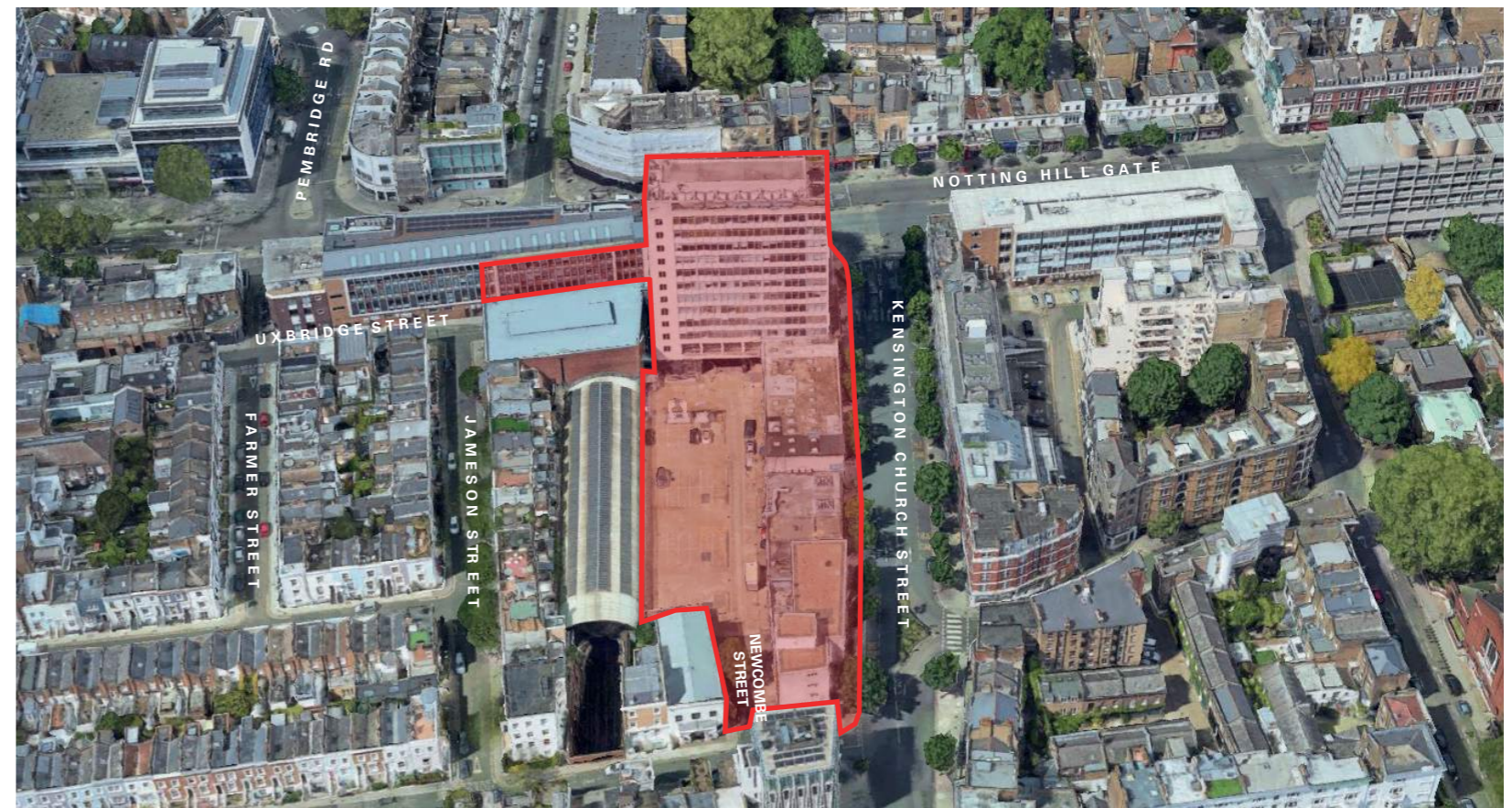
Fig 1.3 - Existing Site looking north
