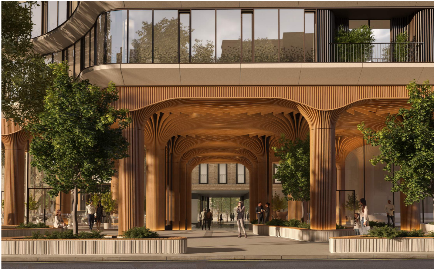
Fig. 3.31: Illustrative view of the double storey entrance and public realm fronting Notting Hill Gate
