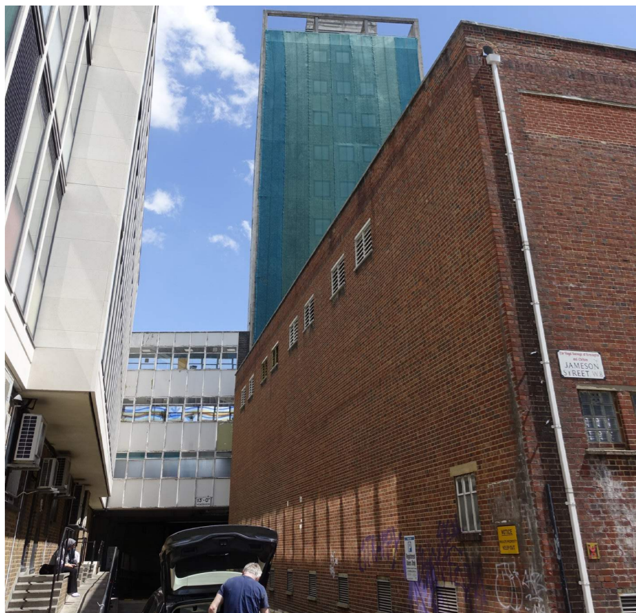
Fig 2.7: View of existing Newcombe House and link corridors from Uxbridge Street
