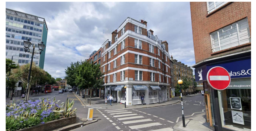
Fig. 3.97: Corner Mansion Block Condition: Kensington Church St. and Kensington Mall
