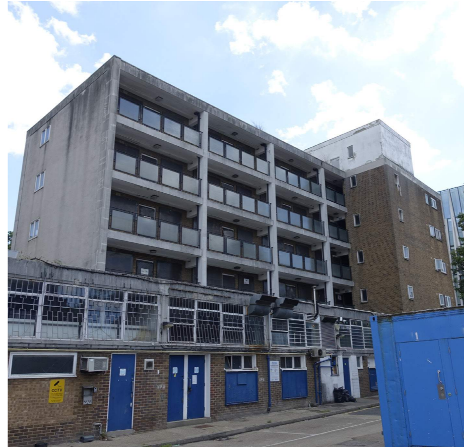
Fig 2.14: View of existing Royston Court rear elevation from carpark
