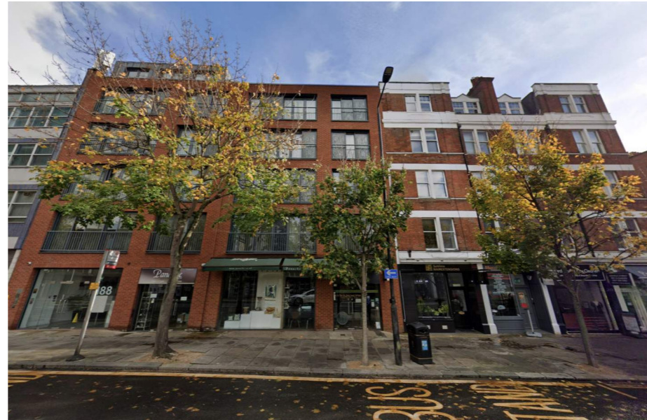
Kensington Church St: Architectural expression of ground floor use and residential above
