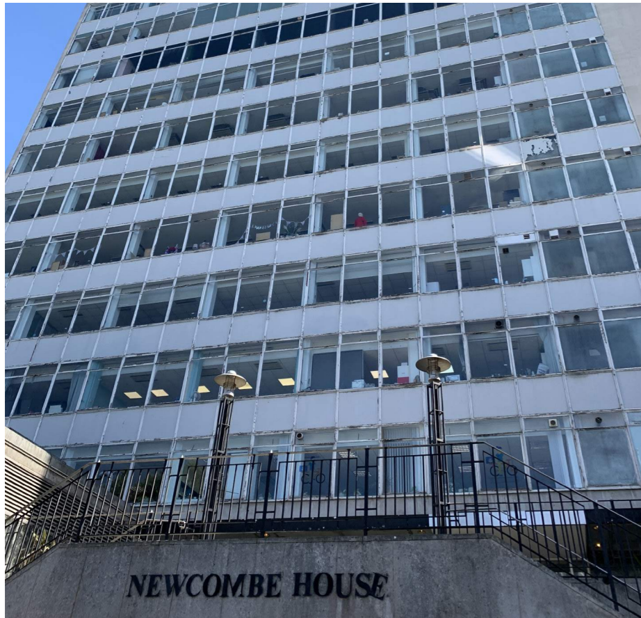
Fig 2.5: View of existing Newcombe House north facade and entrance podium
