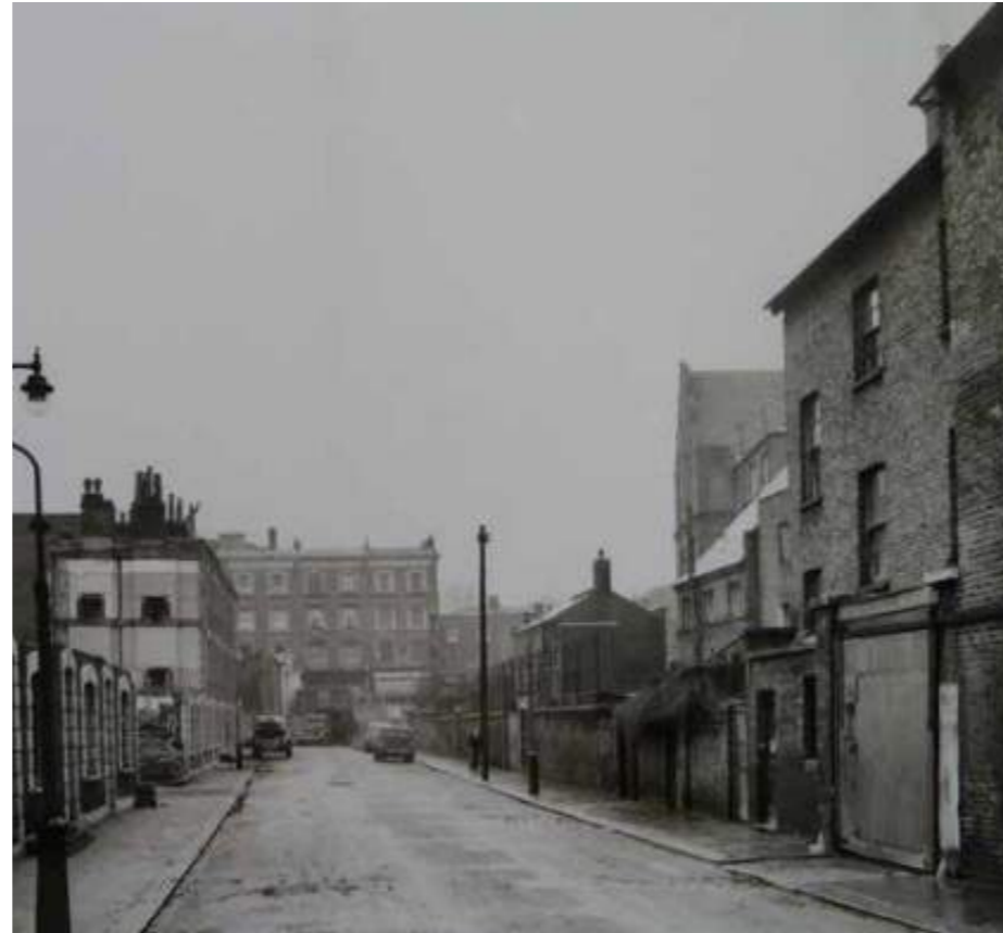
Fig 2.25: Late 1950s photograph of partly demolished terraced houses to Newcombe Street
