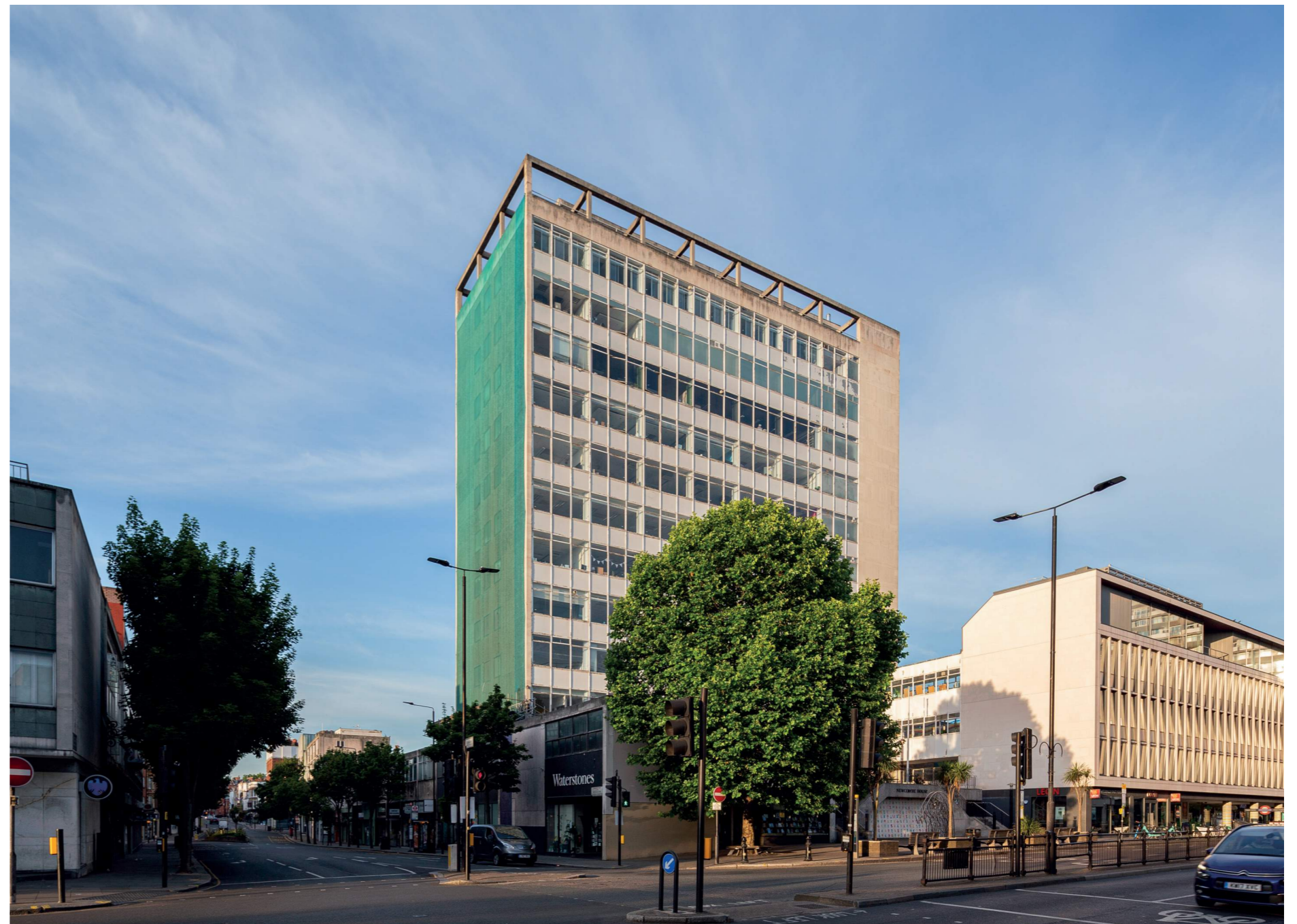
Fig 1.1 - View looking south of the existing site from Notting Hill Gate
