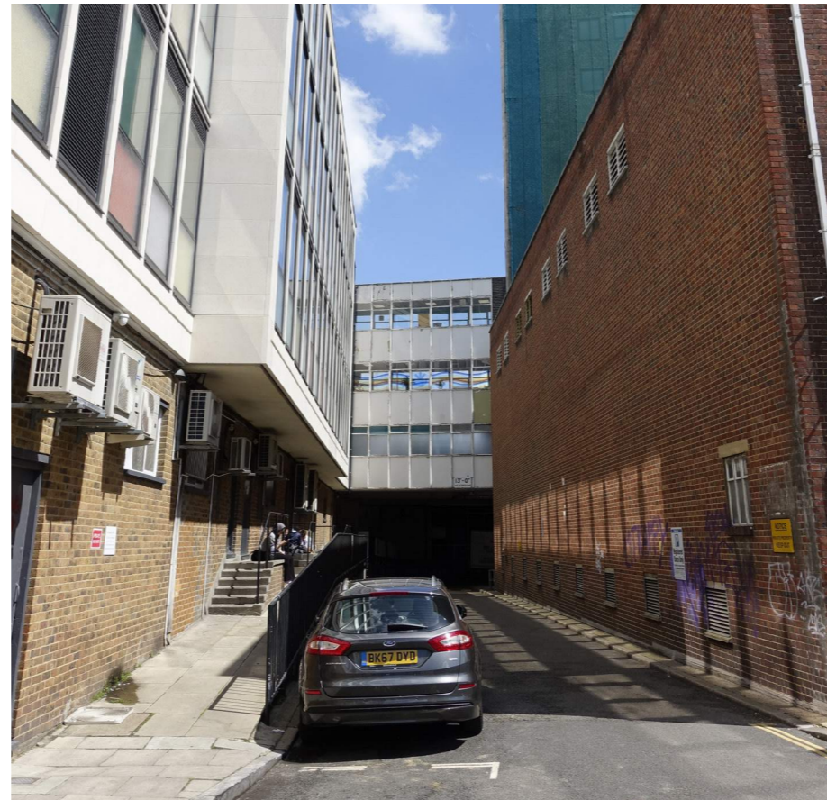
Fig 2.20: View of existing Uxbridge Street and undercroft to Newcombe House beyond
