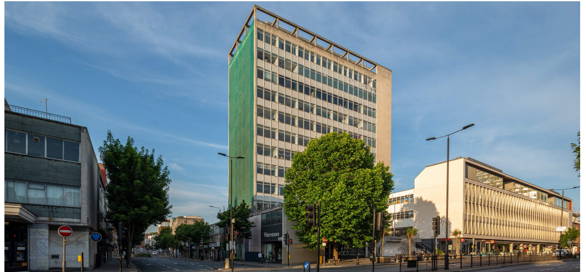
Fig 2.3: View of existing Newcombe House and poor public realm fronting Notting Hill Gate
