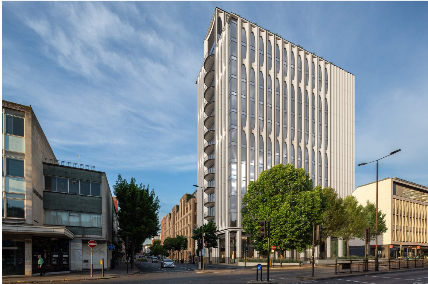
Illustrative view of the Proposed Development with the reduced balcony proposals in context
