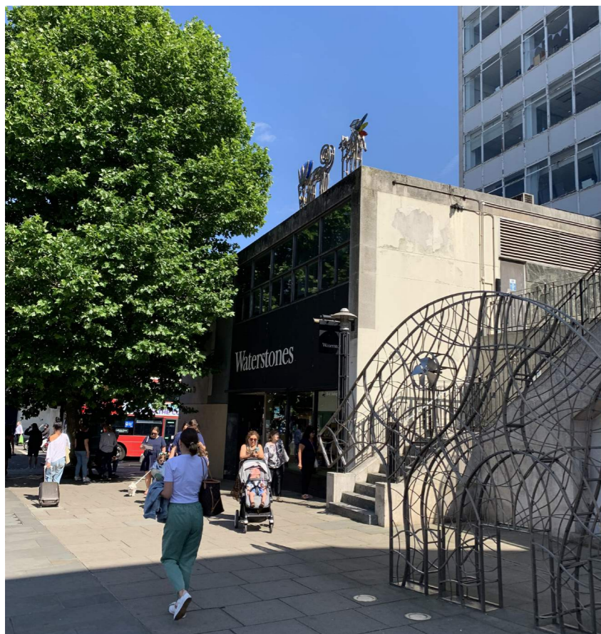
Fig 2.9: View of existing Waterstones corner retail unit to Notting Hill Gate
