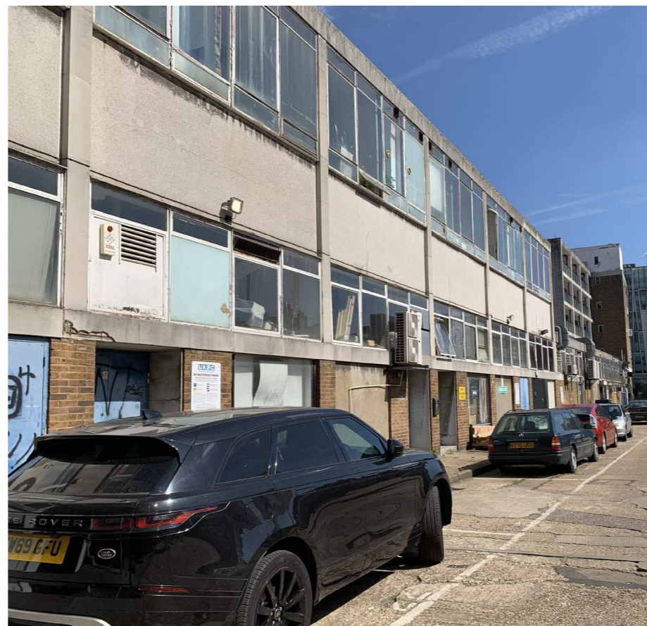
Fig 2.11: View of existing rear facades to the retail units from the private carpark
