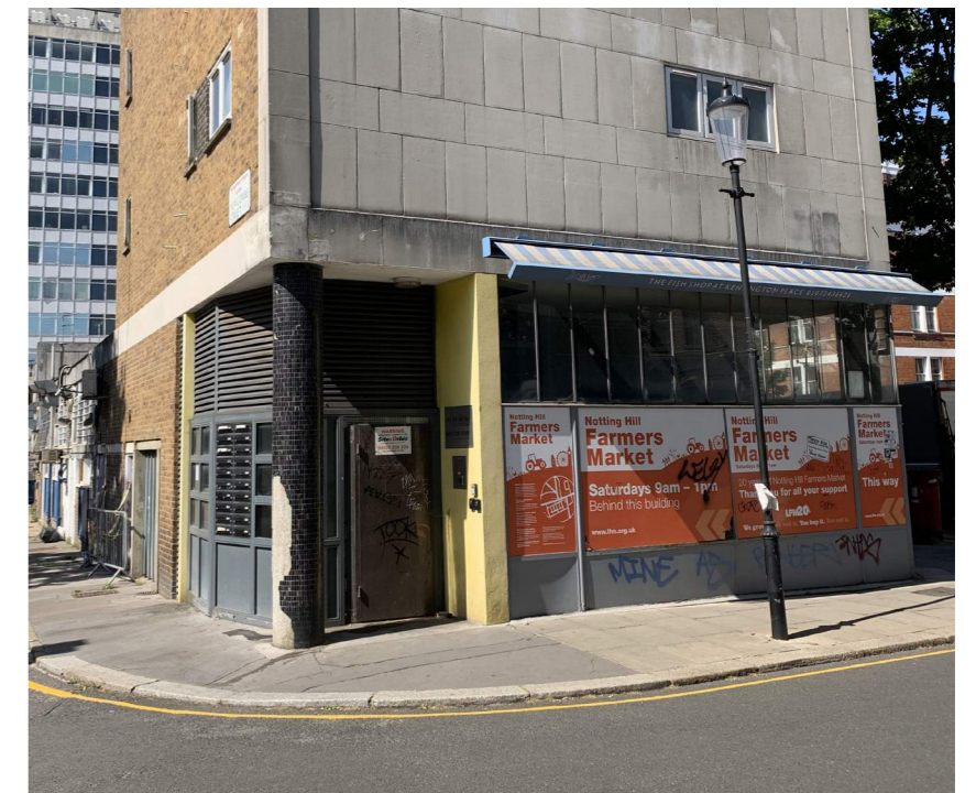
Fig 2.16: View of the existing entrance into Royston Court from Kensington Place
